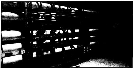
BRINE WATER RECOVERY SYSTEM
